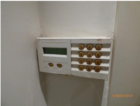
Paint marks to alarm panel
