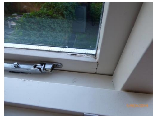
Cracking to window woodwork
